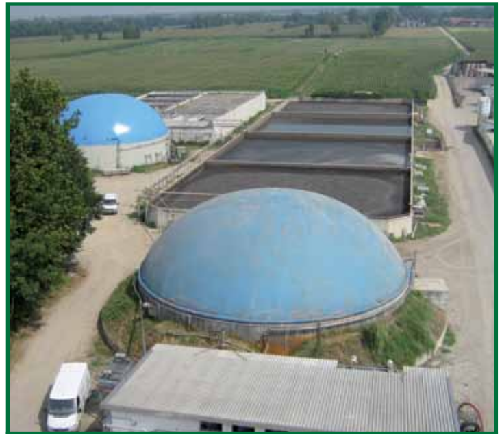
Fitted directly to the top of Anaerobic Digester tanks
