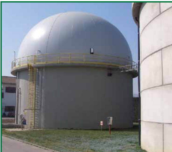
Replacement of existing steel Gas Bells
