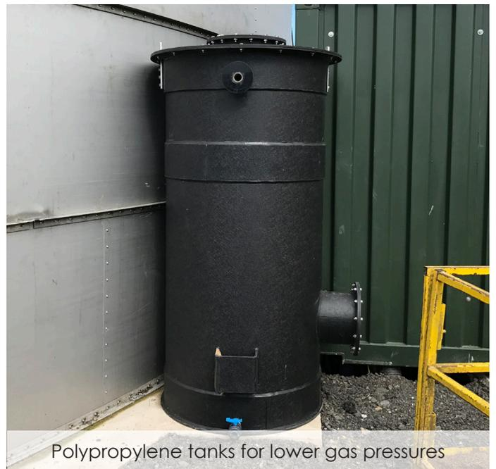
Polypropylene tanks for lower gas pressures
